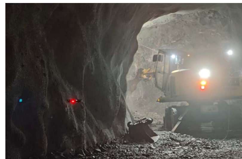
FIG 33 Drone flying inside the Kemi mine during the scaling operation.
