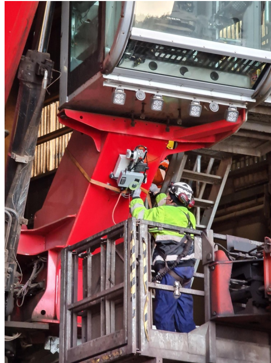
FIG 27 Mounting the portable sensor system on the material handler
